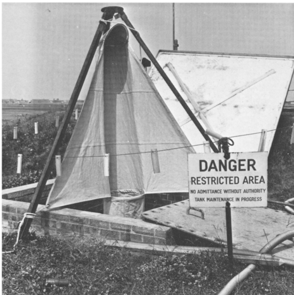
Fig. 3. Wind sail air scoop.
